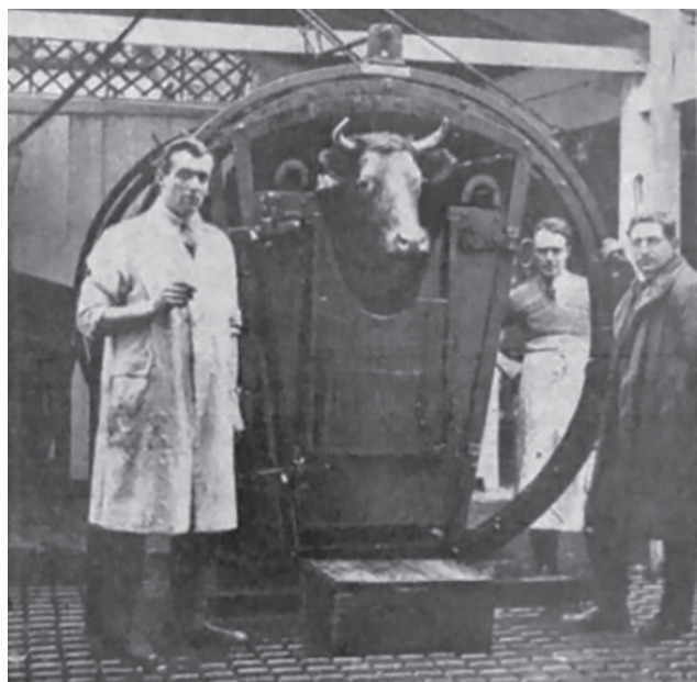
Figure 2: One of the first rotating pens, the “Weinberg” pen, presented in Holland in 1928. Mr. H. Weinberg appears in the picture, on the left, with black overcoat (16).
